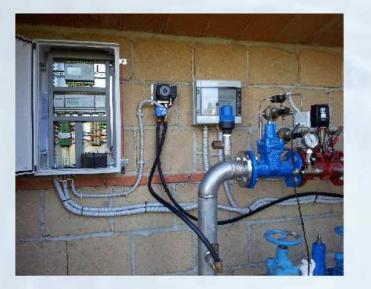
management of regulation and hi/lo pressure valves. Other functions can be inserted on customer request.
